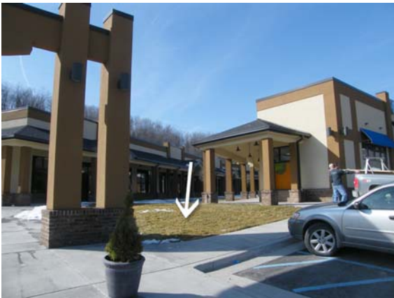
Northwest view from parking lot
