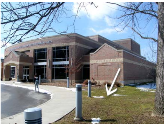
Southwest view - detail
