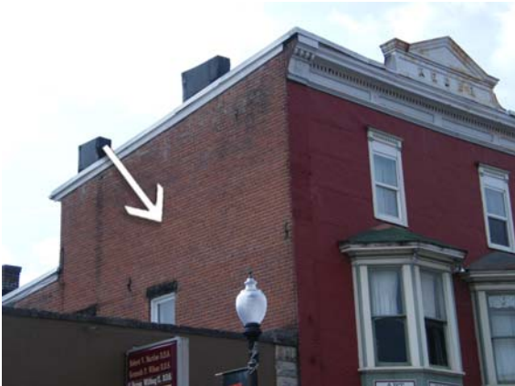
Southwest view – detail
