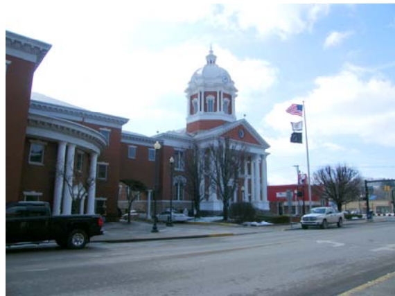
Courthouse view, looking Southwest
